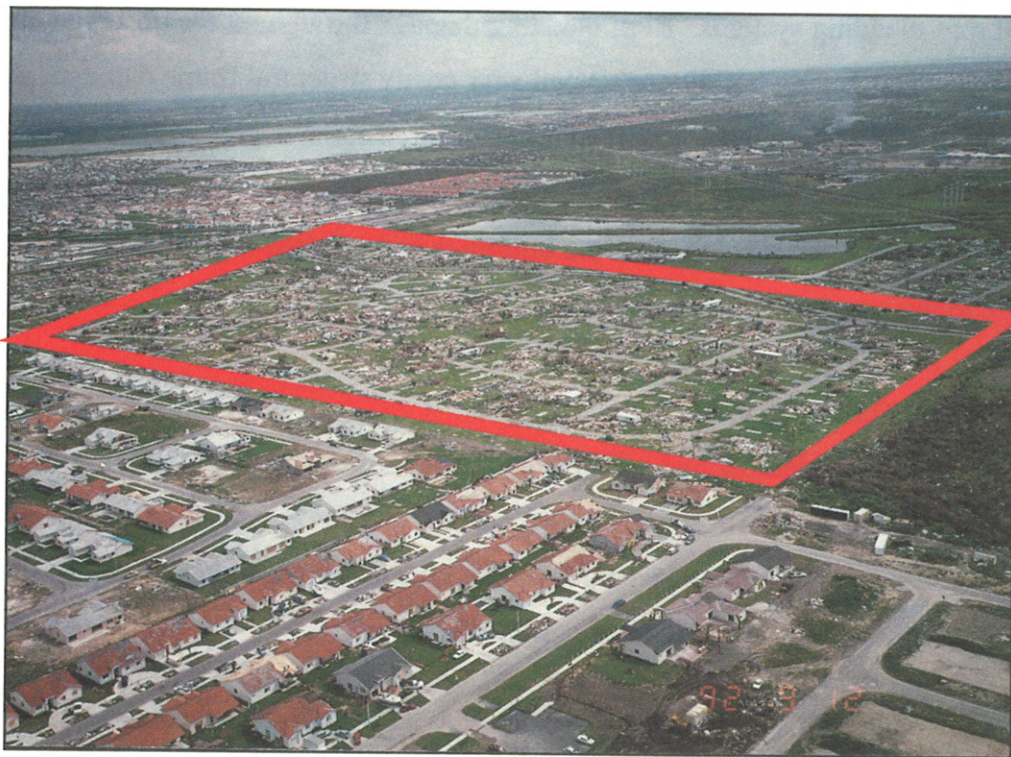
FIGURE 21. Aerial photo of damage area. Shows building performance difference between manufactured homes (outlined in center) and conventional residential buildings (lower left).
